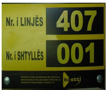
identifier plates shall be fitted on the tee-off tower and on the towers on each side of it. The tower top identifier plate shall identify the circuit and tower number and be fixed on the tower top in such manner that it can be seen from a helicopter.
