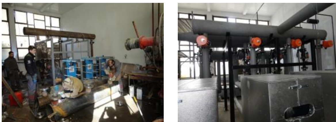
Fig. 6.1 Pictures from the rehabilitation of thermal substation – left, works on reconstruction of the substation; right, substation after the rehabilitation is completed.
